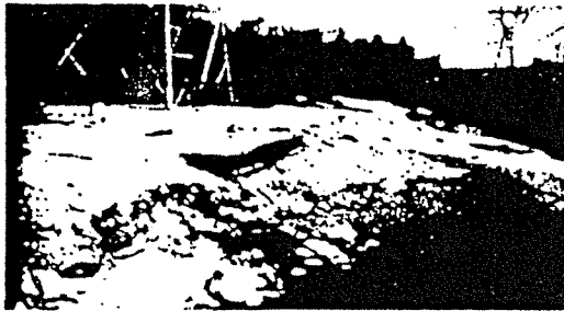
Sheet piling and riprap fail to prevent scour at the base of a 500 kv transmission tower. Raccoon Creek, Paulding County, Ga.
