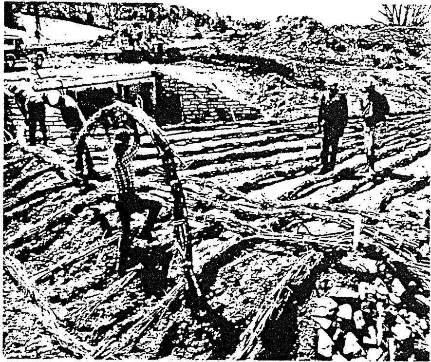
Workers on the Cumberland Gap Tunnel Project site place live fascines (bundles of living plant material) on the live boom, a soil bio-engineering project which is being constructed to redirect the stream of Little Yellow Creek. Alton Simms, (left, background), Vice President of the Soil Bio Engineering Corp., and Barry Carnes, field inspector with Vaughn & Melton, oversee the work.
