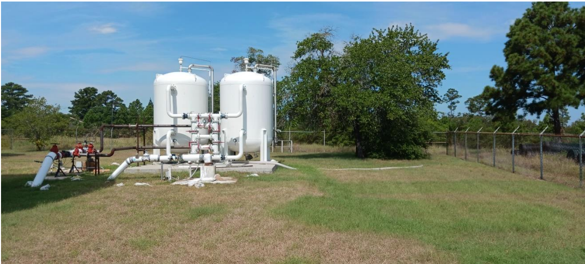
Photo 8 Bastrop County WCID 2 – Water Plant 2, Well 3 and Well 4 Site August 18, 2024
