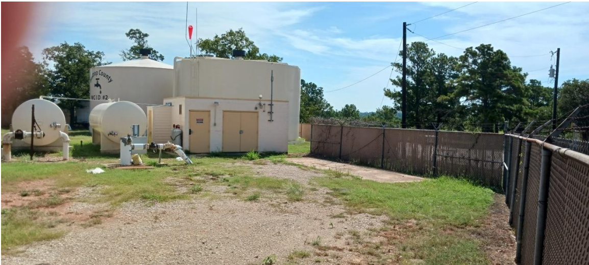
Photo 4 Bastrop County WCID 2 – Water Plant 1, Well 1 and Well 2 Site August 18, 2024
