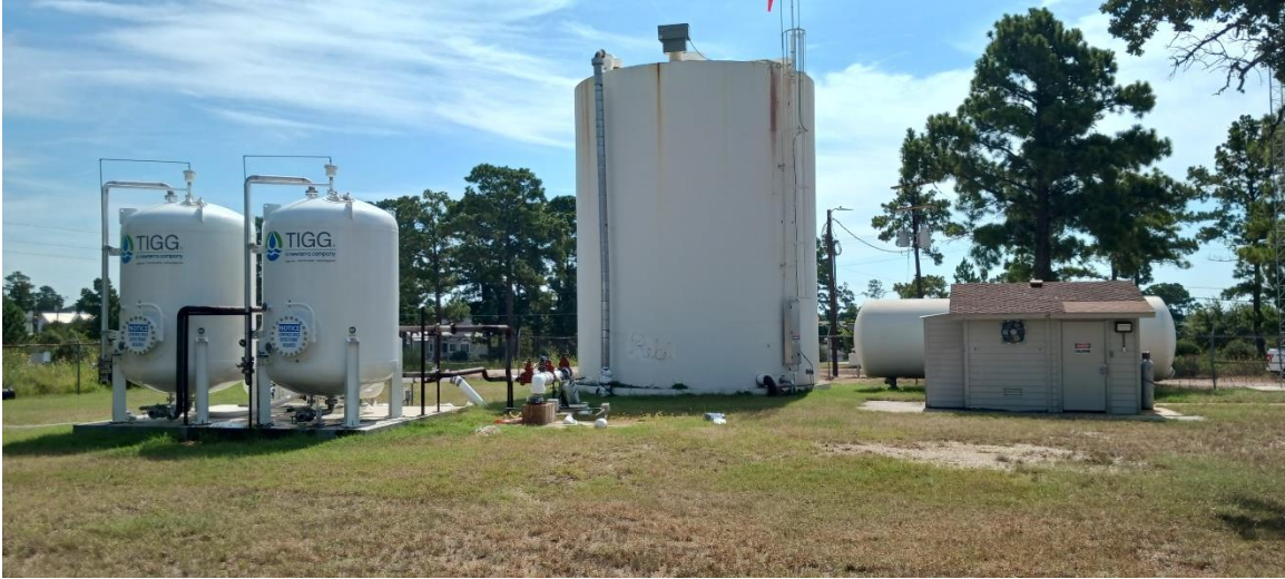
Photo 7 Bastrop County WCID 2 – Water Plant 2, Well 3 and Well 4 Site August 18, 2024
