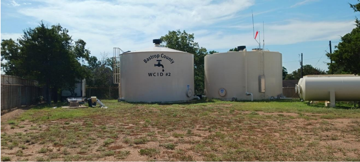
Photo 3 Bastrop County WCID 2 – Water Plant 1, Well 1 and Well 2 Site August 18, 2024
